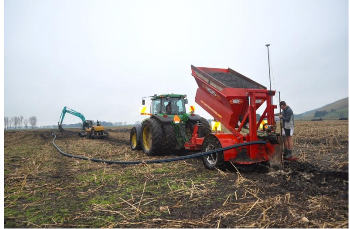
Installing sub-surface drainage with gravel envelope
