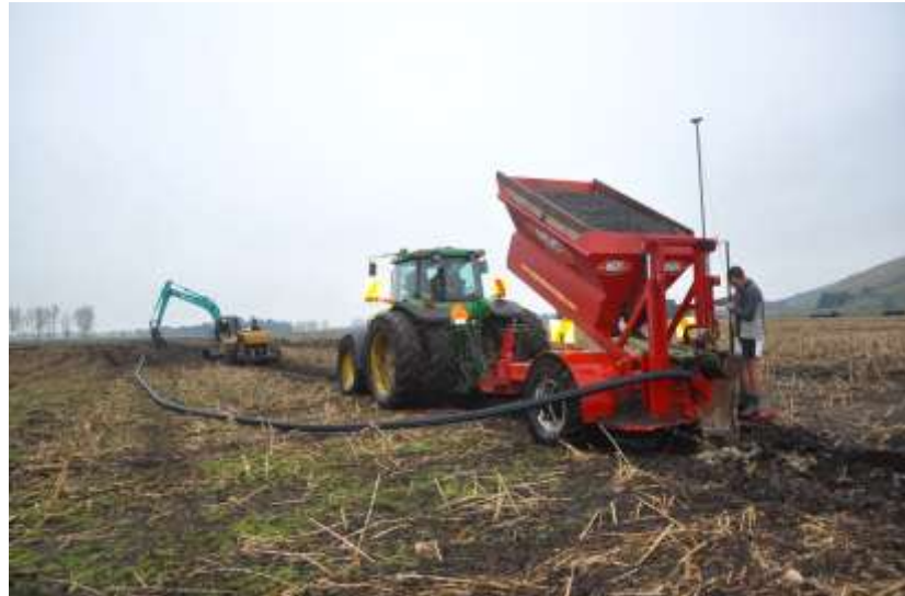
Figure 1 Precision drain layer in action (D. Dixon image)
