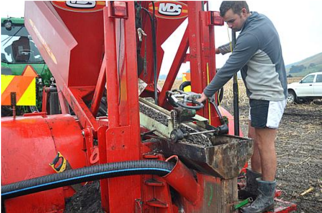
Gravel backfill is laid around drainage pipe (Duke Dixon image)
